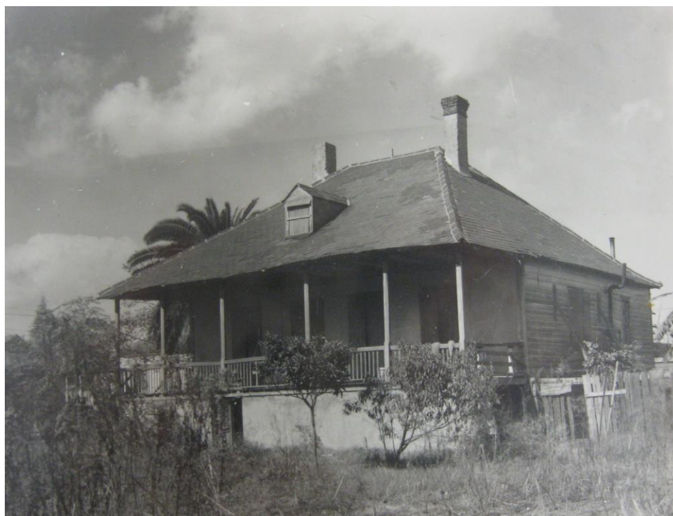
Figure 6 619 Congress Street, photograph 1930s by Richard Koch, Southeastern Architectural Archive, Tulane University.
